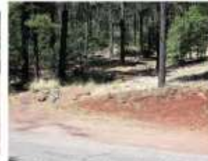
Existing drainage infrastructure on Isabel St
