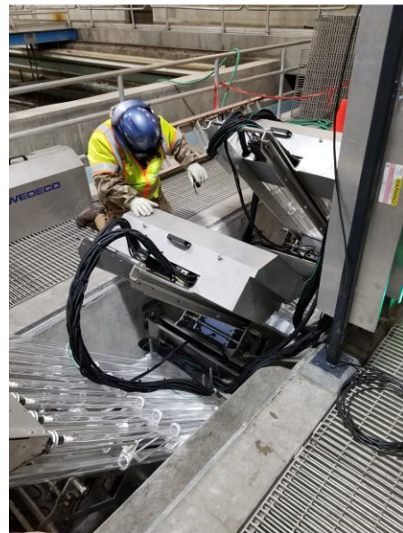
A worker installs the new equipment.
