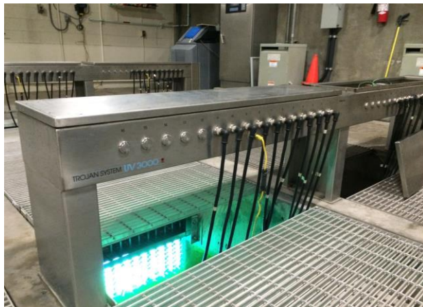
The outdated system was removed.
