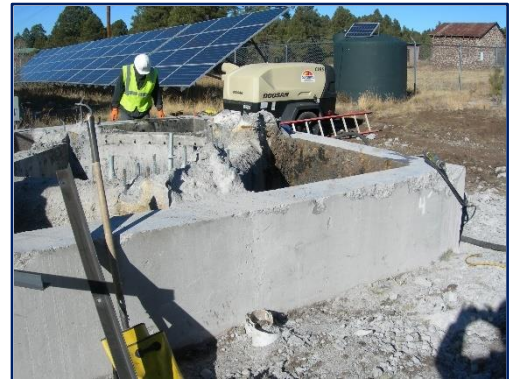
Crews restore the influent structure.
