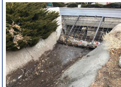
Staff clear the channel to reduce the risk of flooding (after).
